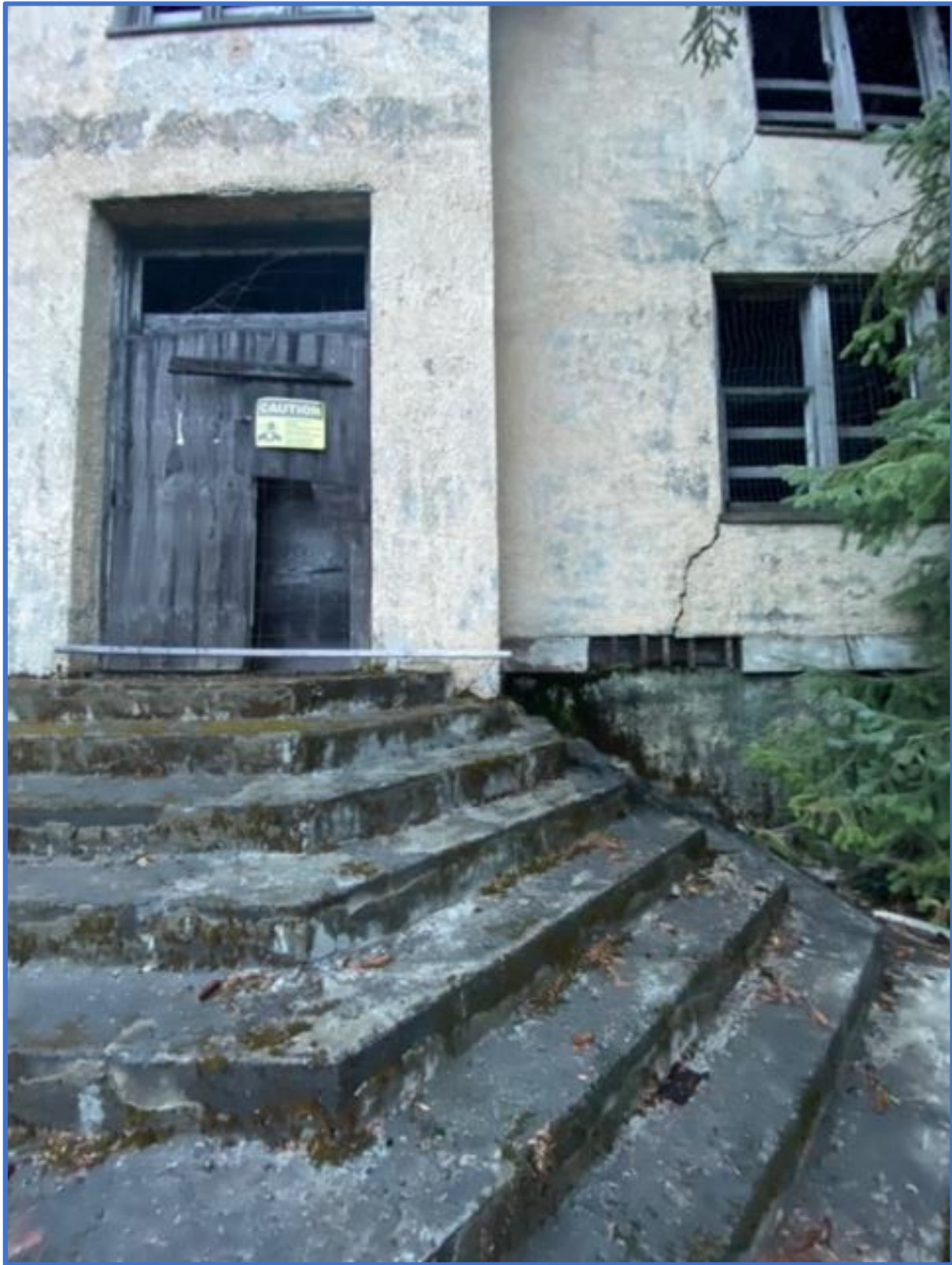
West Stairs of Jesse Lee Home Seward Photograph #1525
