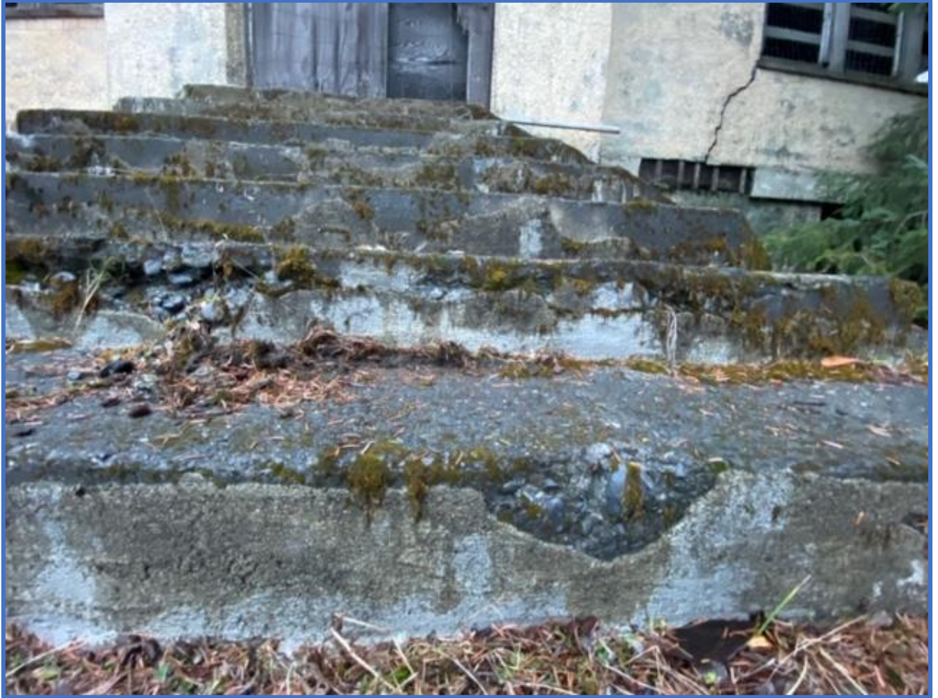
West Stairs of Jesse Lee Home Seward Photograph #1532
