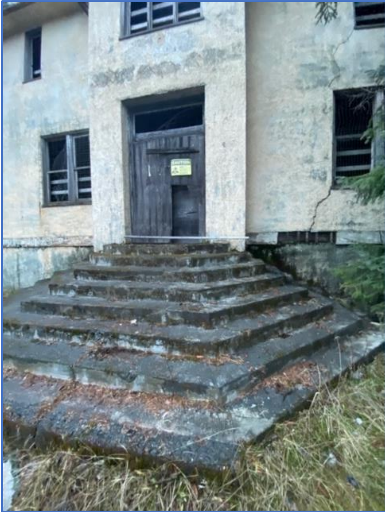
West Stairs of Jesse Lee Home Seward Photograph #1524
