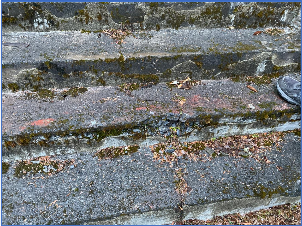
West Stairs of Jesse Lee Home Seward Photograph #1508
