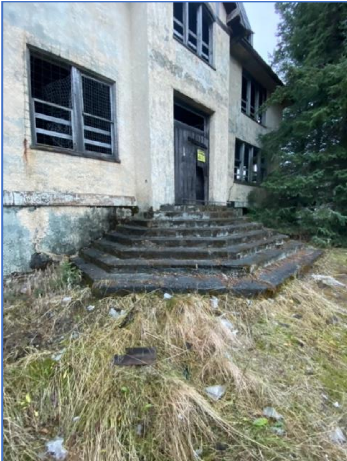
West Stairs of Jesse Lee Home Seward Photograph #1528
