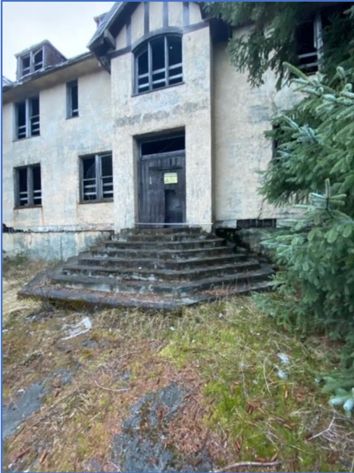
West Stairs of Jesse Lee Home Seward Photograph #1522
