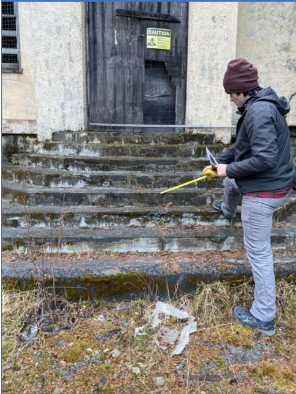
West Stairs of Jesse Lee Home Seward Photograph #1510
