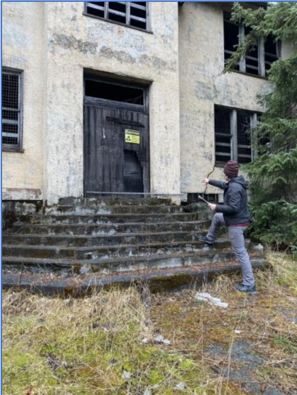
West Stairs of Jesse Lee Home Seward Photograph #1507
