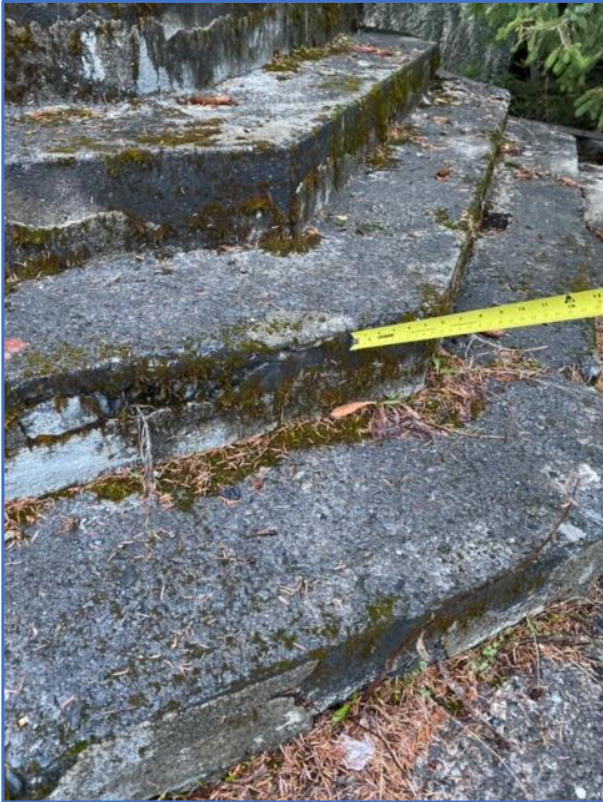
West Stairs of Jesse Lee Home Seward Photograph #1512
