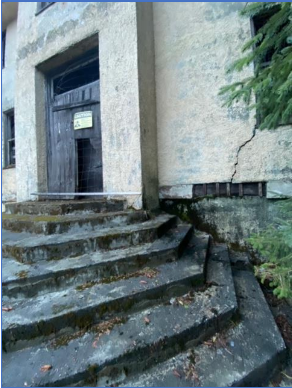
West Stairs of Jesse Lee Home Seward Photograph #1526
