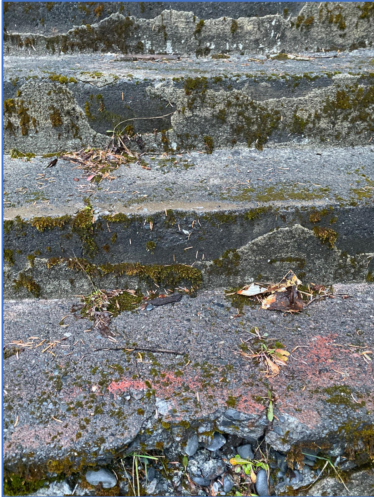
West Stairs of Jesse Lee Home Seward Photograph #1509
