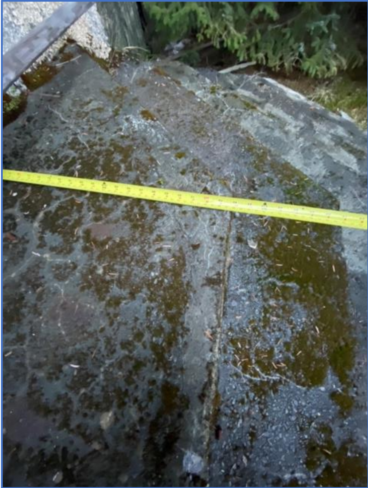
West Stairs of Jesse Lee Home Seward Photograph #1517
