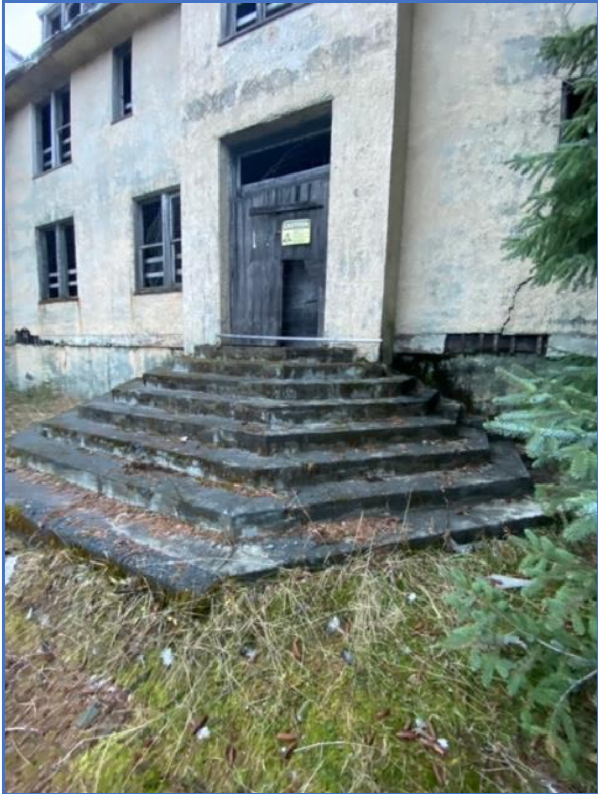
West Stairs of Jesse Lee Home Seward Photograph #1523
