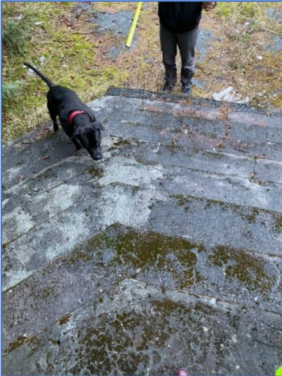
West Stairs of Jesse Lee Home Seward Photograph #1511
