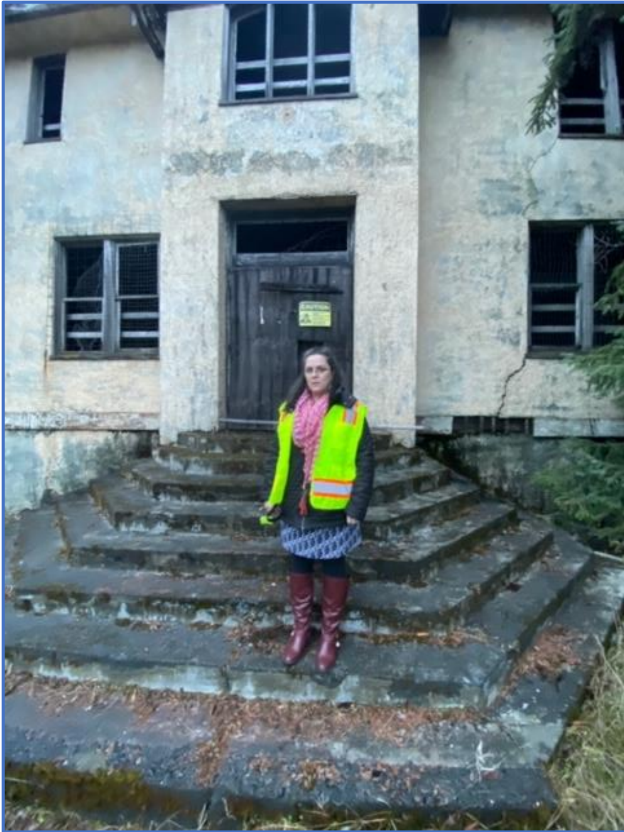
West Stairs of Jesse Lee Home Seward Photograph #1519
