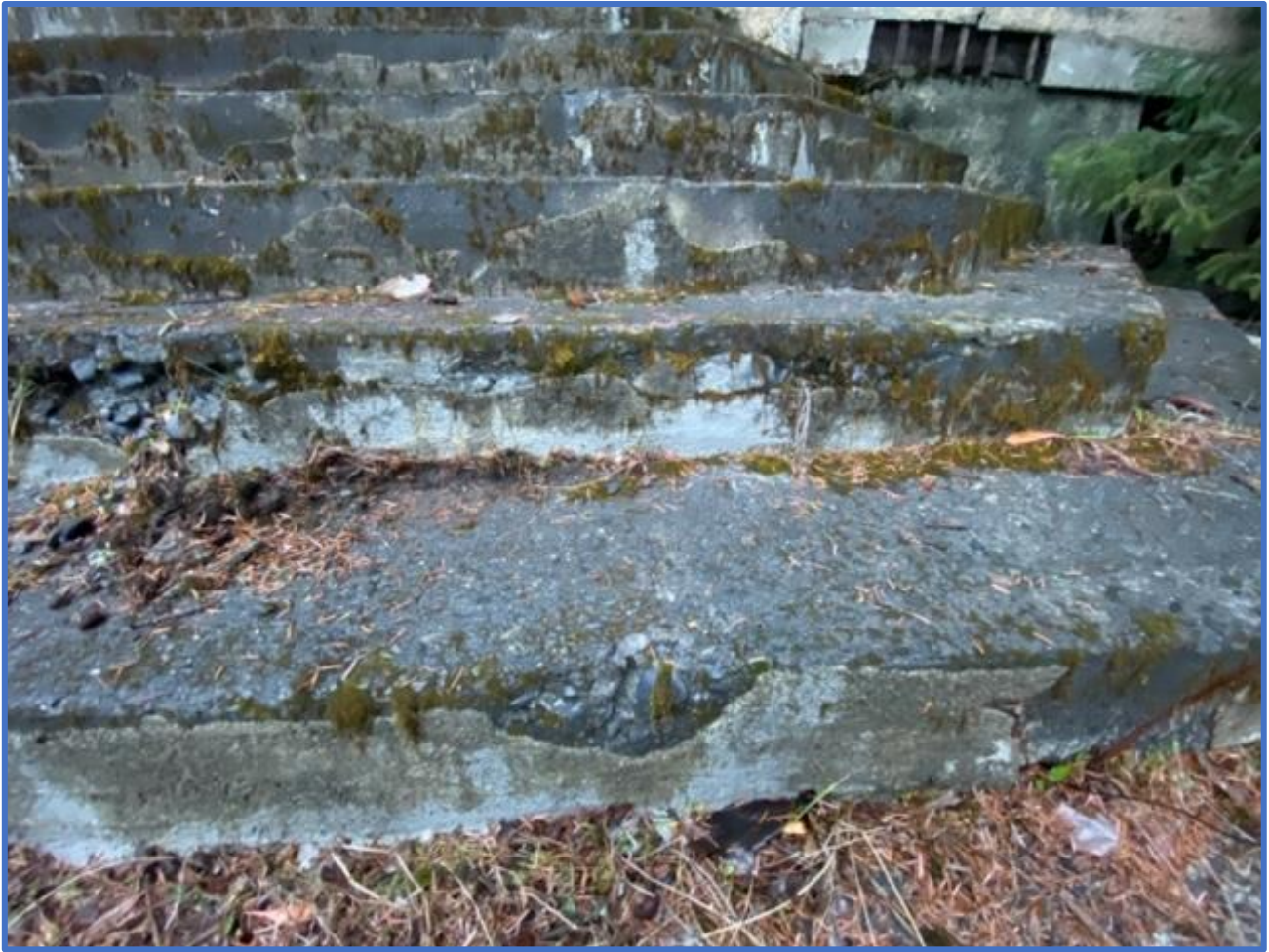
West Stairs of Jesse Lee Home Seward Photograph #1533
