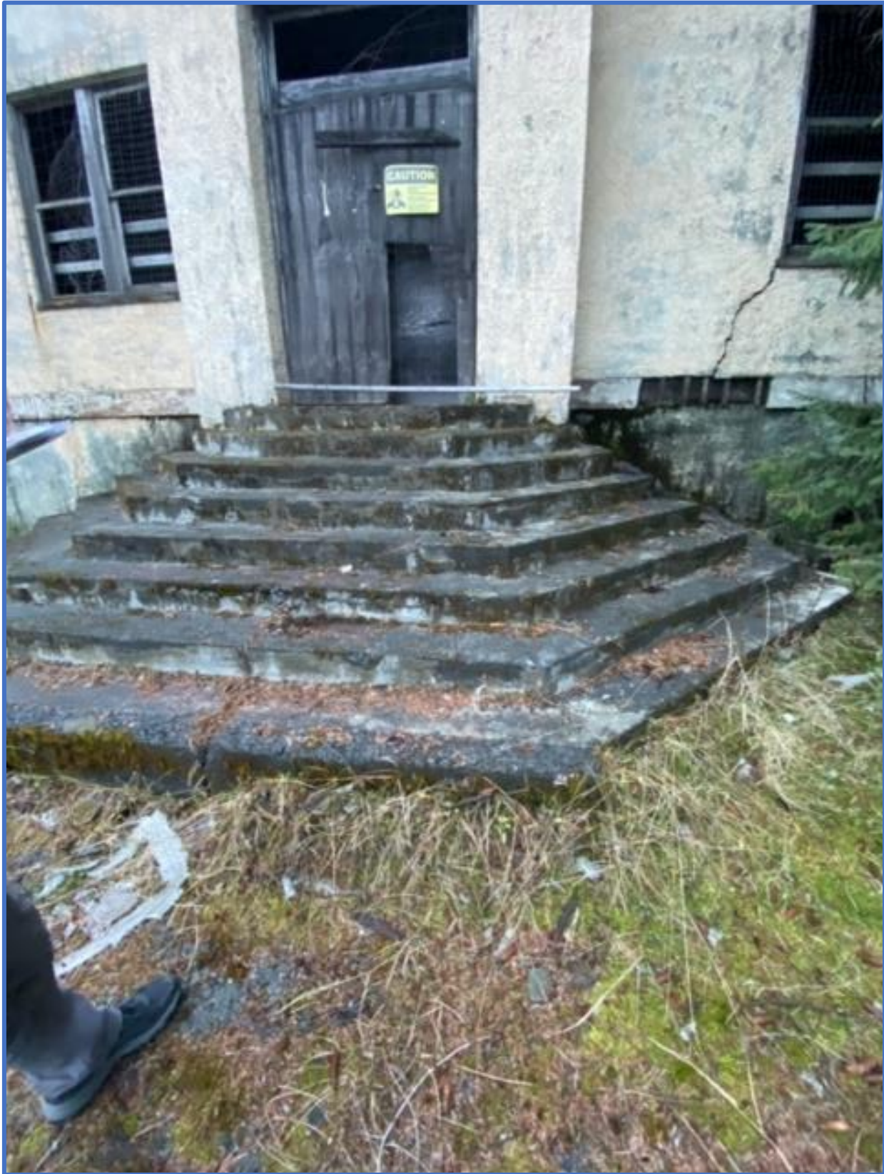
West Stairs of Jesse Lee Home Seward Photograph #1527
